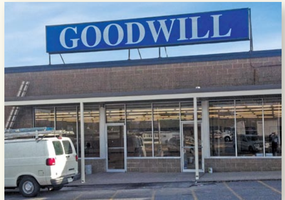
Final work being done in preparation for Verona store's January opening.
